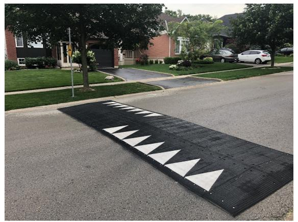
Figure 2: Temporary Speed Hump Example
