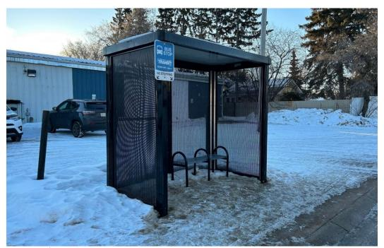
Figure 2: 15<sup>th</sup> Avenue East Transit Shelter with Perforated Metal Panel Installation. Shelter glass was 75% replaced in 2022. The remaining shelters will have laminated glass or perforated metal panels installed in 2023 to further improve rider comfort.
